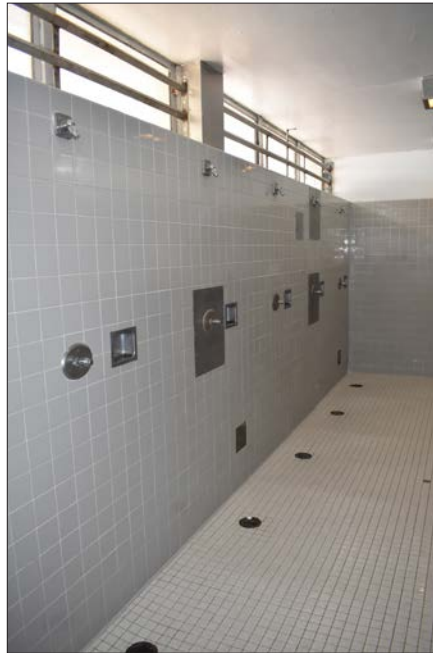
Figure 19. Photo of Showers in Barracks
